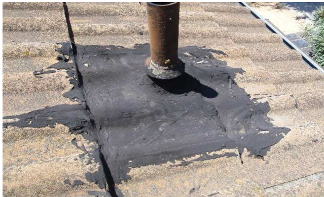
Shingles containing Mastic (typically around chimneys or pipes)
